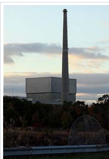
Oyster Creek Generating Station in Lacey Township
